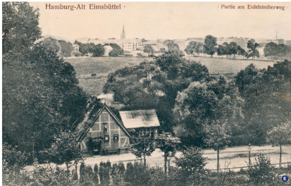
Top: View from the first Beiersdorf factory of what is today Unnastraße in the direction of the Apostelkirche church, circa 1900 Bottom: Topping-out ceremony for Troplowitz's private house and the factory building behind it in 1892
